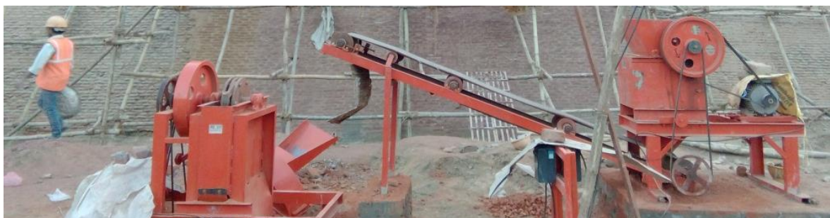
Figure 4: Showing Grinding Machine process of making Surkhi
