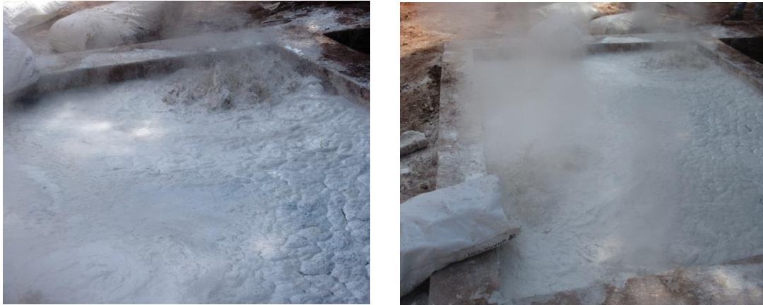
Figure 2: showing the Slaking Process of Lime
